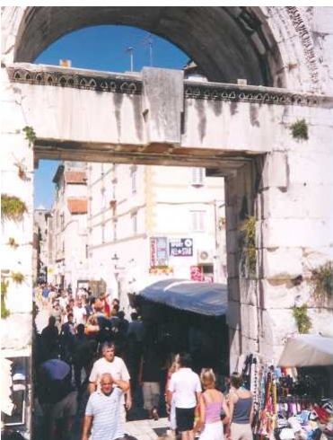
Split, Croatia: East Gate—a flat arch
