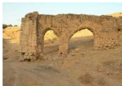
Ottoman period Aqueduct to grain mill
